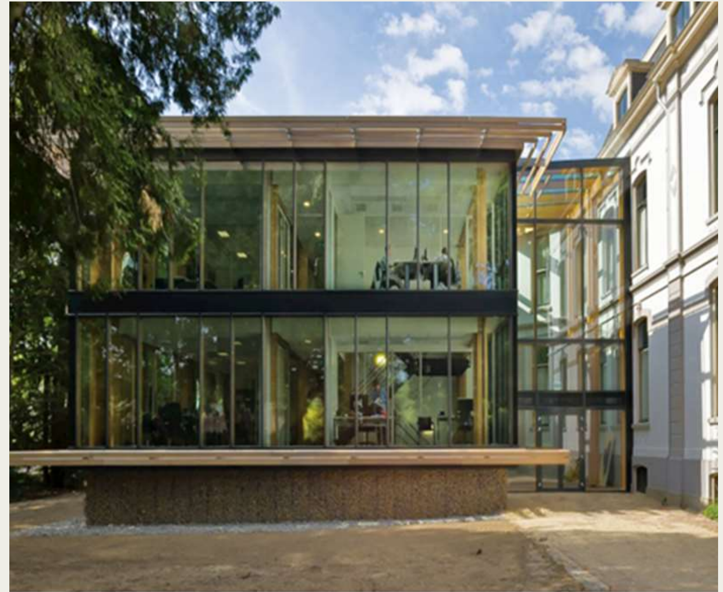
Brummen Townhall, The Netherlands is designed for disassembly, where 90% of the materials can be dismantled and reused.
